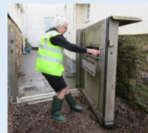
Lympstone flood warden operating flood gate
