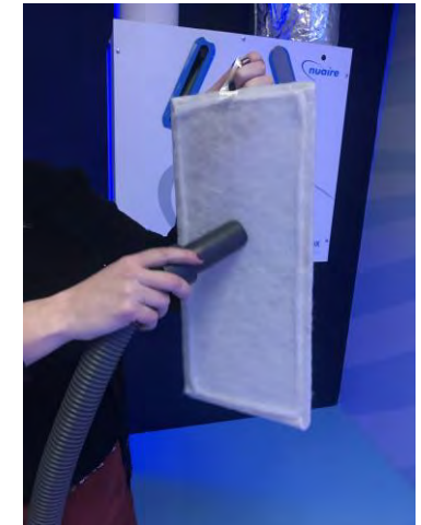
MVHR filters are easy to remove and clean, clean filters improve energy efficiency. (Sources: Vent Axia, Nuaire,)
