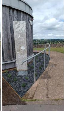
The wooden handrail on the ramp beside the Canal Tea Rooms and Garden has been deteriorating in recent years with some small sections of timber rotting. It was not possible to find a matching handrail and so rather than replacing just the rotted section, the Canal Ranger Service had to replace to whole 40m length.
