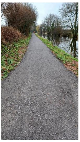
Near Halberton, a section where the path had been worn down to the liner – between Crownhill Bridge and Tiverton Road Bridge - has been resurfaced as shown above right.
