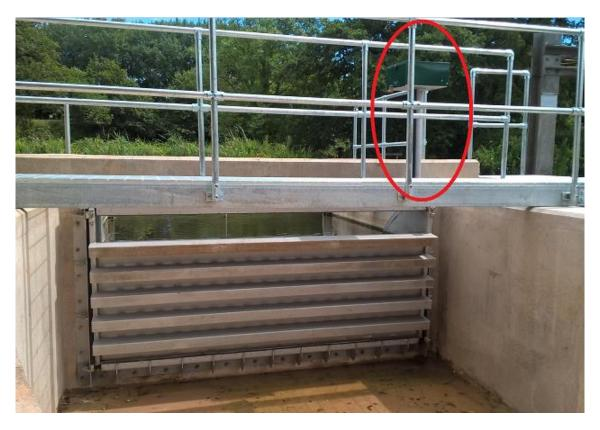
The 3m tilting 'door' is controlled by a 'Greenbox' (circled red above) which incorporates the motor, gears, batteries, solar panel, electronics and transmitter/receiver for receiving commands and sending updates via the website portal. The Greenbox and website portal was supplied and maintained by a Dutch company which has recently lost a major contract in the Netherlands and has folded as a result.
