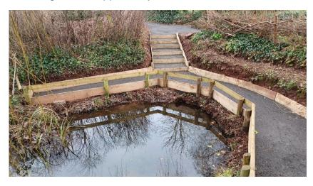
water level. To make it easier and safer, we engaged an excavator contractor to dig down the standing level by 30cm. The Canal Rangers and volunteers then edged the paths, built new steps and used crushed stone to resurface all around, including the main path through the garden which had been becoming increasingly puddly.
