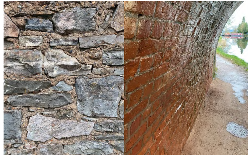
Left, stone walling, right English bond brickwork
