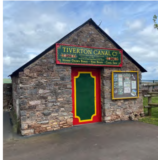
Tiverton Canal Company beside the canal
