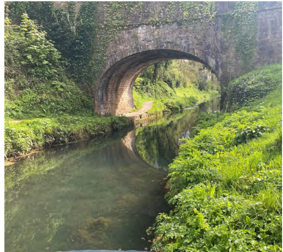
View of the canal beside Whipcott Bridge
