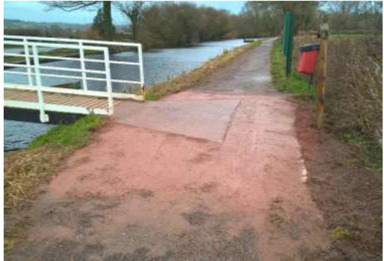
After being scraped off, the towpath beside the offside end of the Dudley Weather Jubilee Lift Bridge was resurfaced to bring it up to the same level as the concrete pad, which had begun to stand proud and create a trip hazard.
