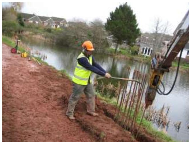
5. When all 260 steel rods were fully inserted over the 20m length, the trench was filled back in and the area was made good (right).
