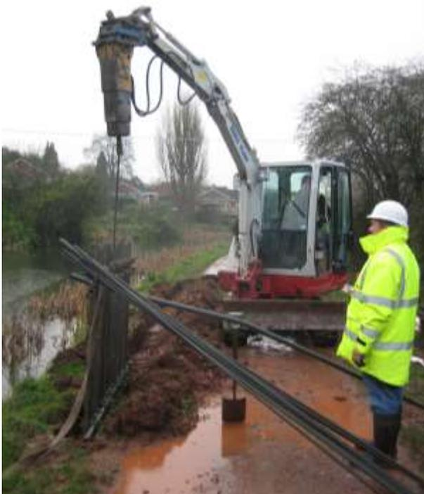
3. One by one the frame tubes were loaded with steel rods and these were pushed in by the excavator (only a few actually needed the hydraulic action of the 'pecker' to hammer them in the required depth) (left).
