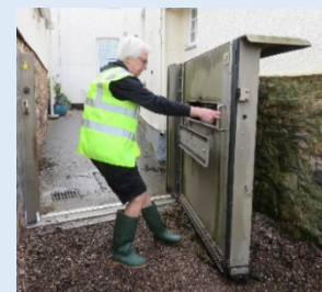
Lymestone flood warden operating flood gate
