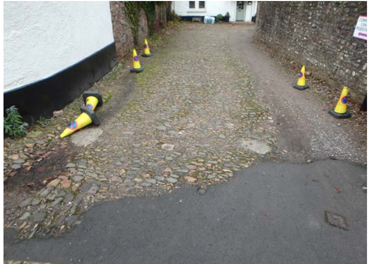
Cobbles at Pye Corner showing damage.
