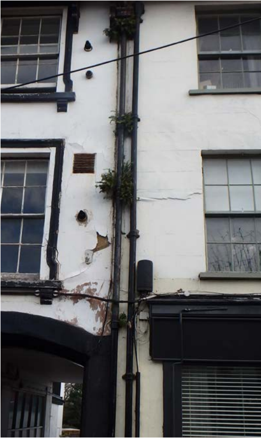
Blocked and overflowing downpipe
