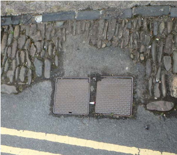
Cobbles damaged by utilities on Church Street
