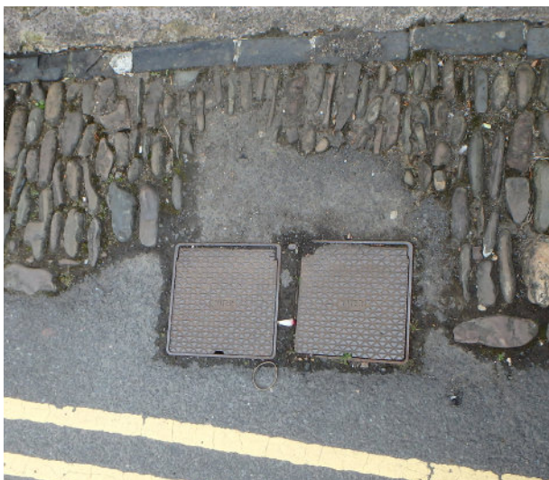
Cobbles damaged by utilities on Church Street
