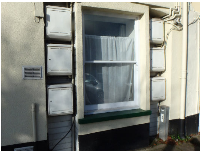
Six utility boxes on front of converted house
