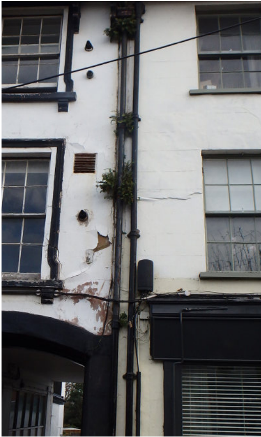
Blocked and overflowing downpipe
