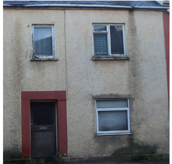
Long term damage from poorly maintained rain water goods
