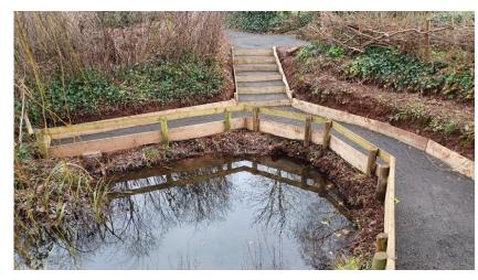
water level. To make it easier and safer, we engaged an excavator contractor to dig down the standing level by 30cm. The Canal Rangers and volunteers then edged the paths, built new steps and used crushed stone to resurface all around, including the main path through the garden which had been becoming increasingly puddly.
