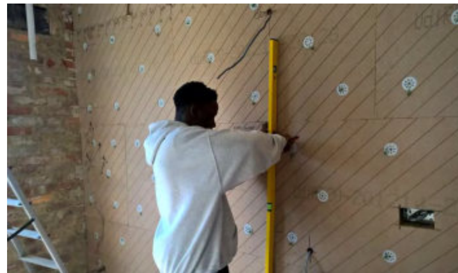
Installation of wood fibre insulation boards internally (Sources Back to Earth & ASBP)
