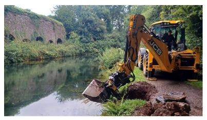
Sealing a leak beside Westcott Bridge using puddling clay
