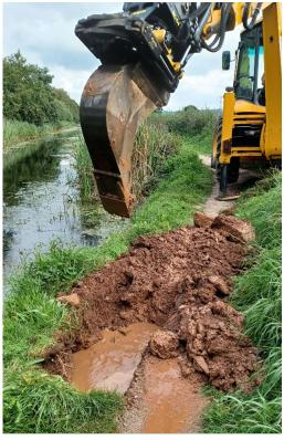
Rebuilding an eroded section of bank beside Manley Bridge.
