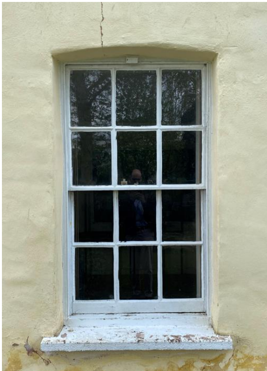
Timber sash window upon Moorings
