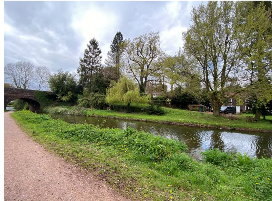
View of Rock House, Rock Cottage and Rock Bridge
