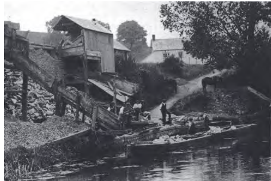
Stone being loaded at Whipcott Wharf
