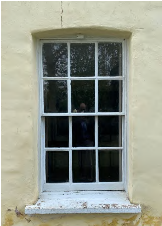
Timber sash window upon Moorings
