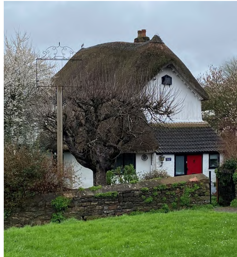
Lime Kiln Cottage
