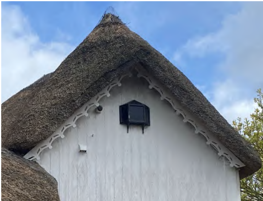
View of decorative barge boards upon Lime Kiln Cottage
