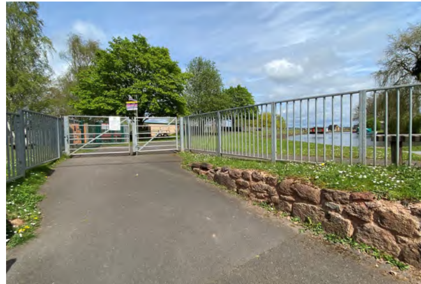
View of railings by Canal Hill
