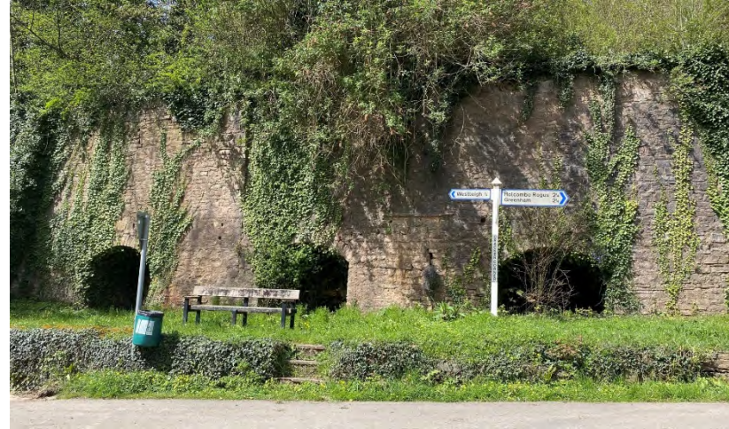
Grade II listed Limekilns at Canonsleigh
