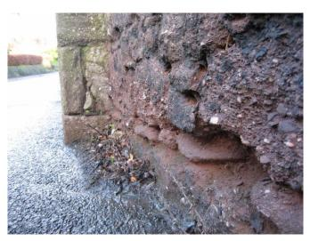
There is also a gradually worsening problem with the wall between the garden of The Moorings and the road. Spray from cars is slowly eroding the soft breccia stone and undermining the wall along the bottom 40cm. Corporate funding has been secured to address this issue by installing a kerb and adding a shoulder of cement to protect the bottom courses of the wall from further erosion. This work will be undertaken whilst the current road closure is in effect in order to avoid further disruption.
